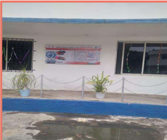
AWARENESS DISPLAY BOARD NR. ADMINISTRATIVE BUILDING
