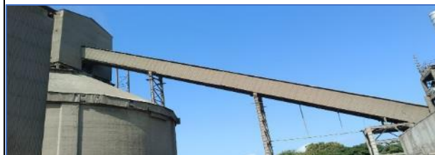
Closed Conveyor belt for clinker
