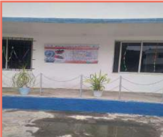
AWARENESS DISPLAY BOARD NR. ADMINISTRATIVE BUILDING
