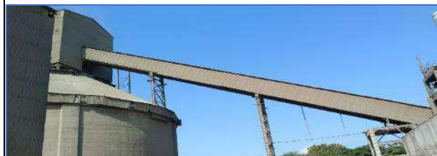
Closed Conveyor belt for clinker
