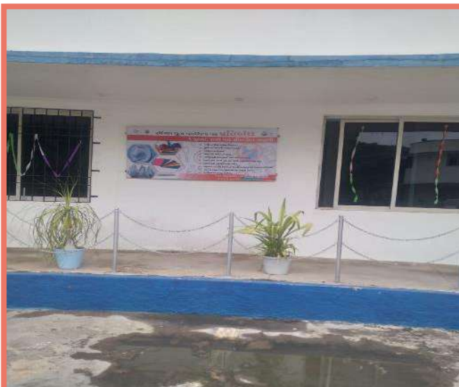
AWARENESS DISPLAY BOARD NR. ADMINISTRATIVE BUILDING
