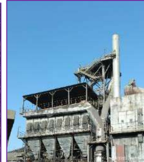
APCM in Raw Mill Bag House & Coal Mill Bag House
