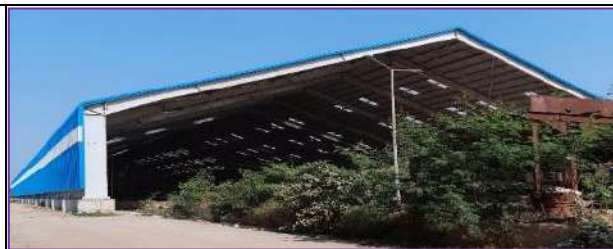
Limestone covered storage Shed
