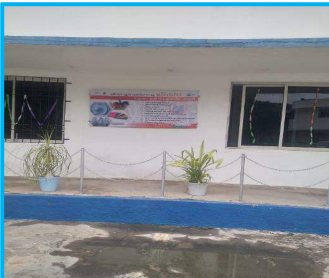
AWARENESS DISPLAY BOARD NR. ADMINISTRATIVE BUILDING
