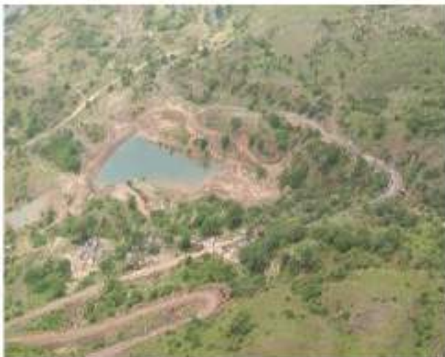
WATER RESERVOIR AT GOP
